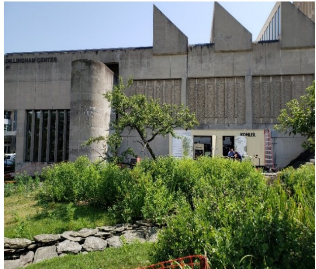
New generator for Peggy Ryan Williams and Dillingham
