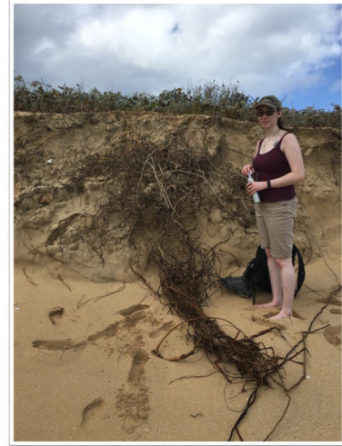
Miranda Ella ('19) surveys storm damage in Culebra over Spring Break 2018.
